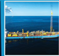
Ships Liquid Cargo Pumping
