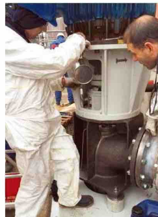
We can appreciate the oil filling phase of the trust bearing chamber, located in the Head Drive of the pumps.
