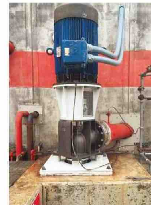
The pump installed, ready for the first start up hydraulic test. This fire-fighting pump works few hours on weekly basis to satisfy the power station safety tests performing every week.
