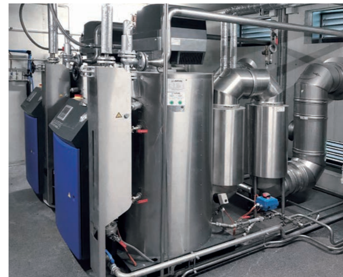
Fig.: Multiple unit steam systems. Second downstream JUMAG economiser installed space-efficiently on the basic frame
