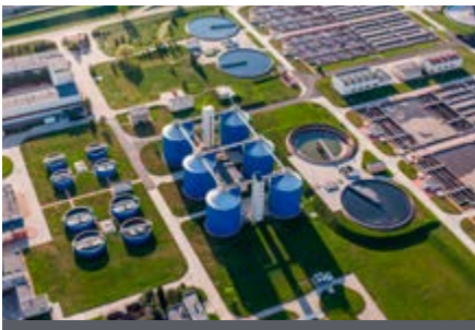
Sewage treatment plants
